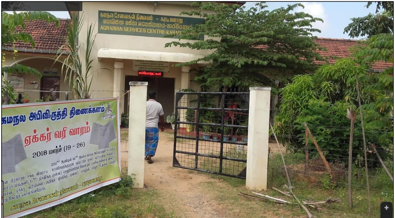
Outside View of ASC Karadiyanaru
